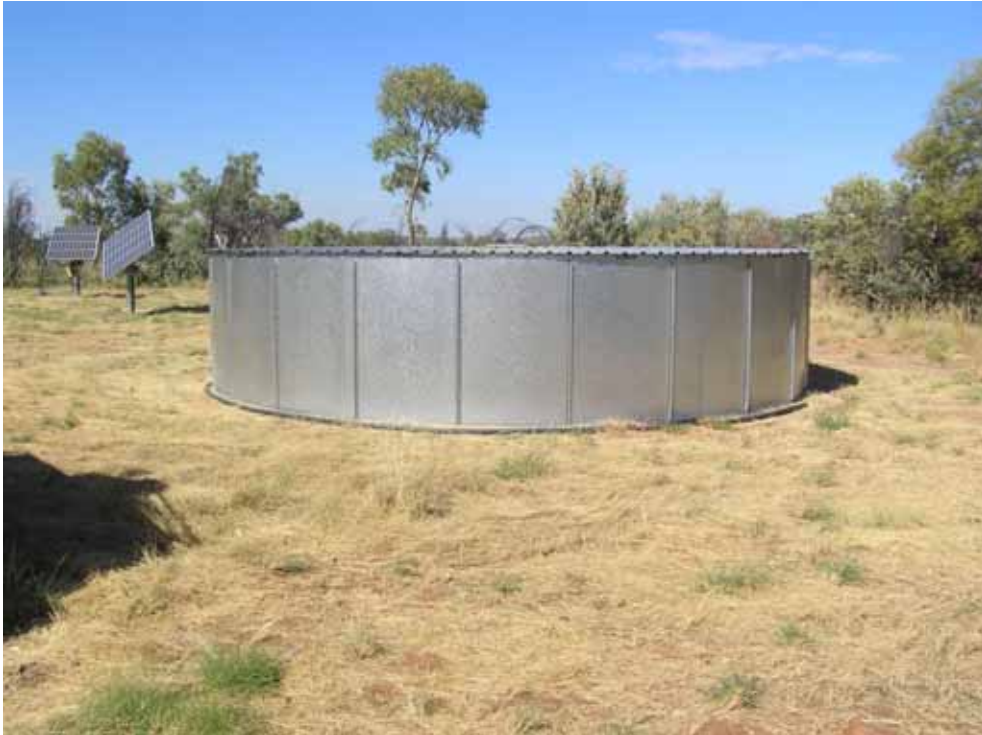
Figure 3. Solar bores (background) and water storage facility
