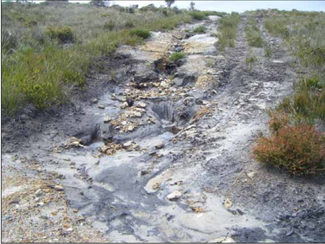
IMAGE 3. ACCESS TRACK EROSION FOLLOWING HEAVY RAINFALL ON MT GARDNER (DEC PHOTO)
