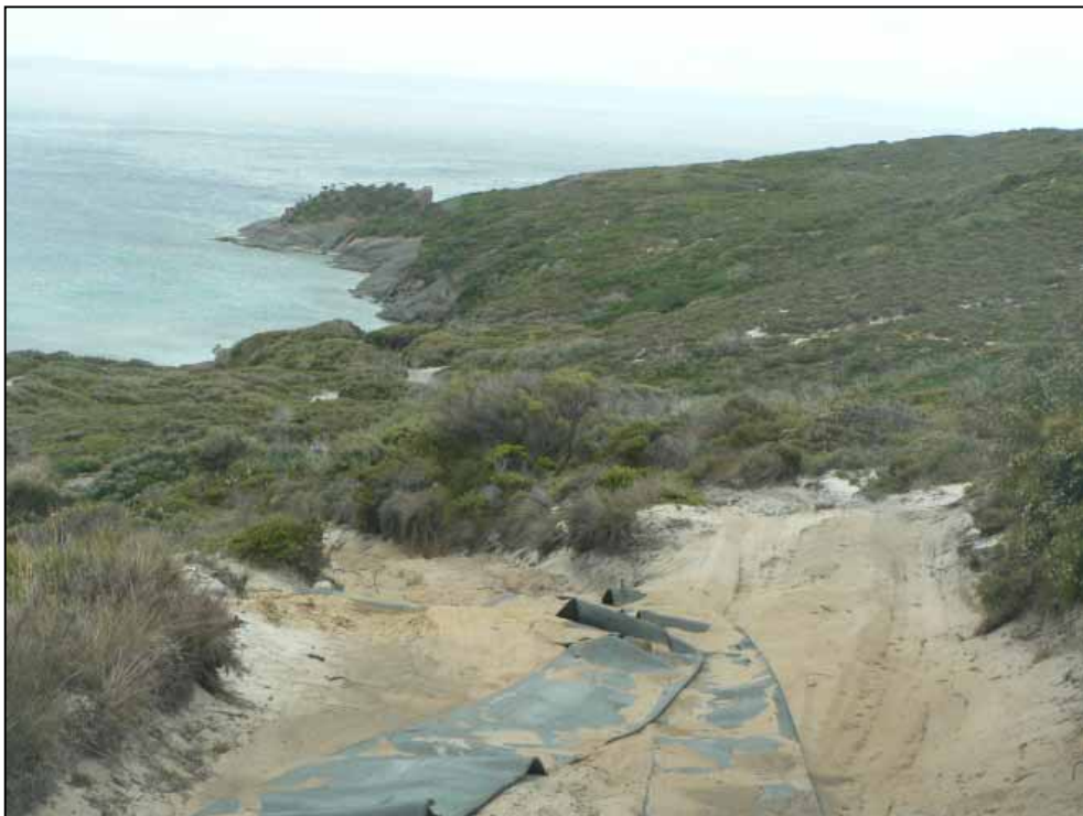
IMAGE 11. ORIGINAL ERODED TRACK TO THE LEFT AND RECENTLY OPENED PUSH THROUGH TRACK TO THE RIGHT
